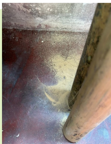
Figure 10. Defective bamboo logs with powdery dust from bamboo holes after insect infestation © Chuen Mun Wai
