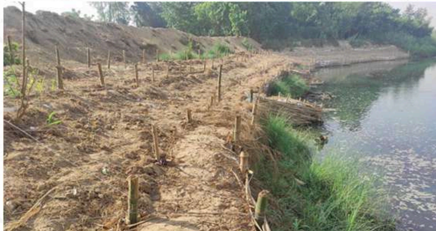
Under construction in 2022
